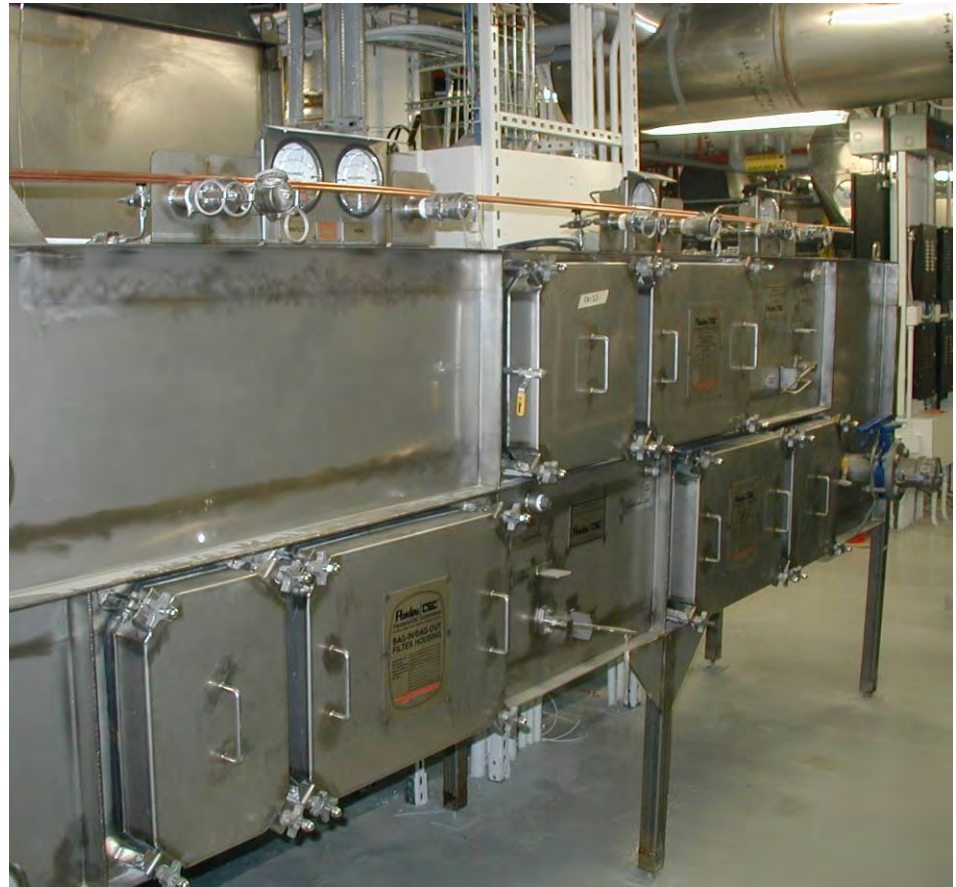
Bag-in, bag-out HEPA filtration caisson
