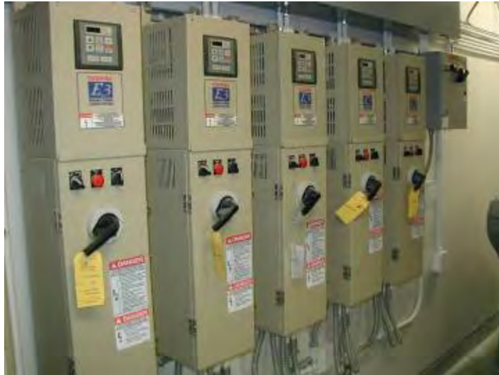
VFD Exhaust Drives
