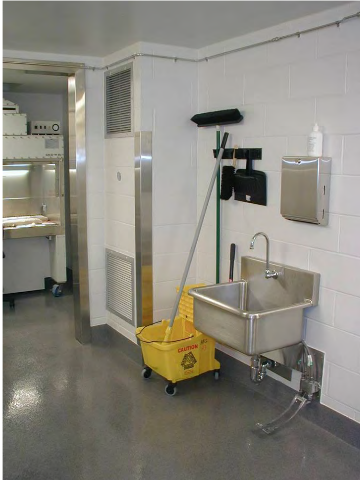
ARC Sink – Utility Station
