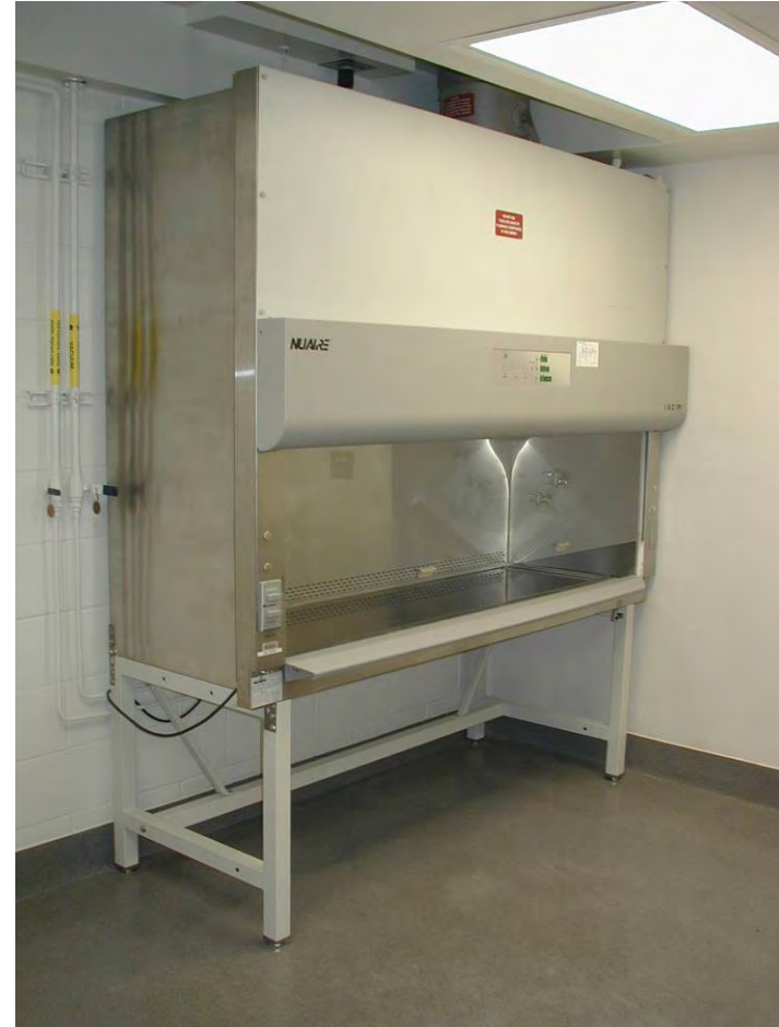
Raised Ceiling for BSC installation
