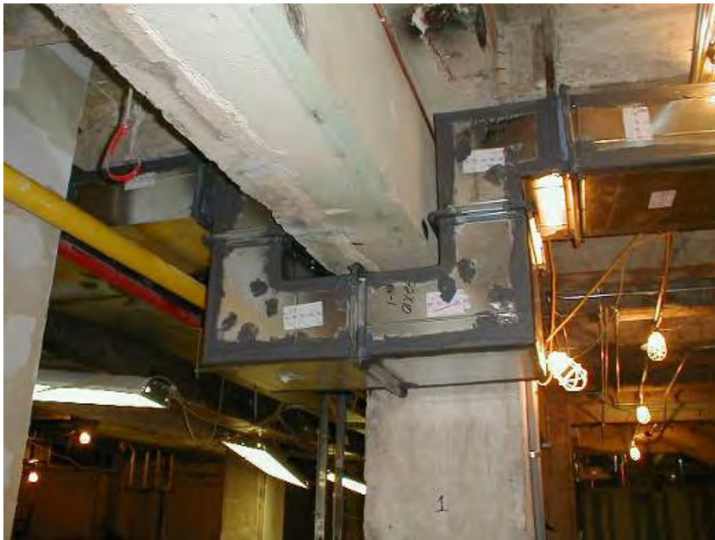
Low Headroom, Limitations due to Existing Structure, Equipment Coordination
