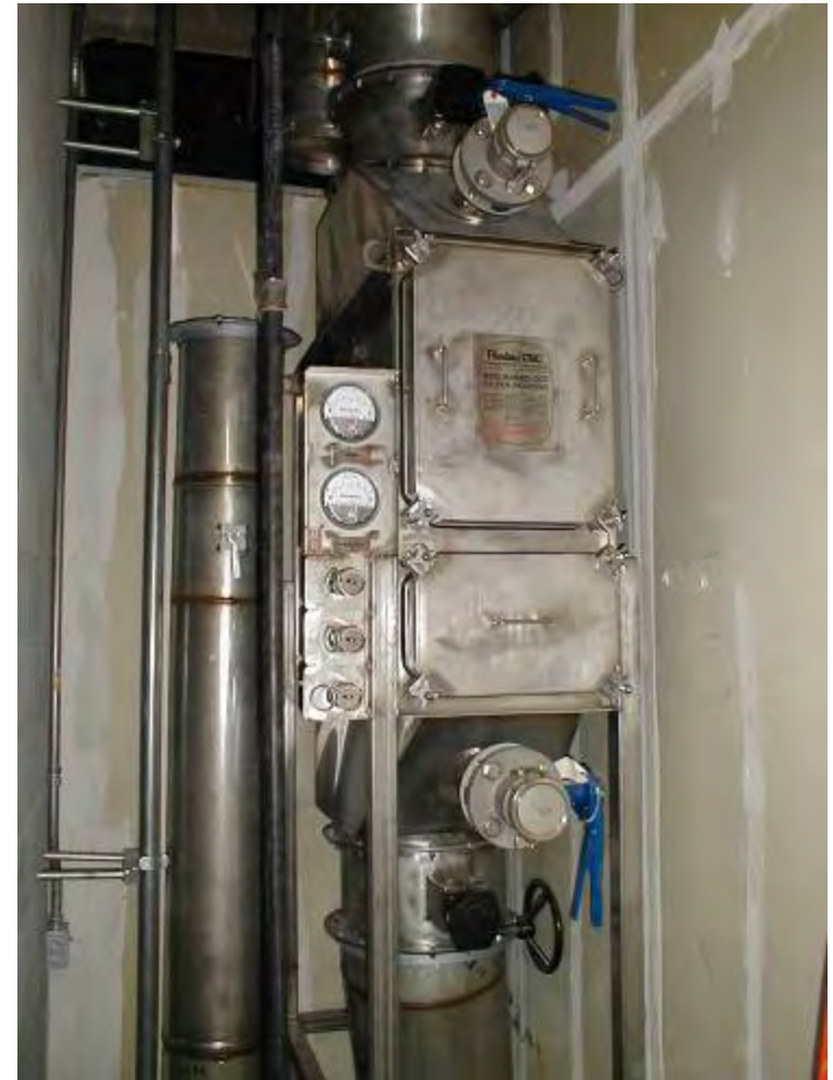
Exhaust manifold in service closet
