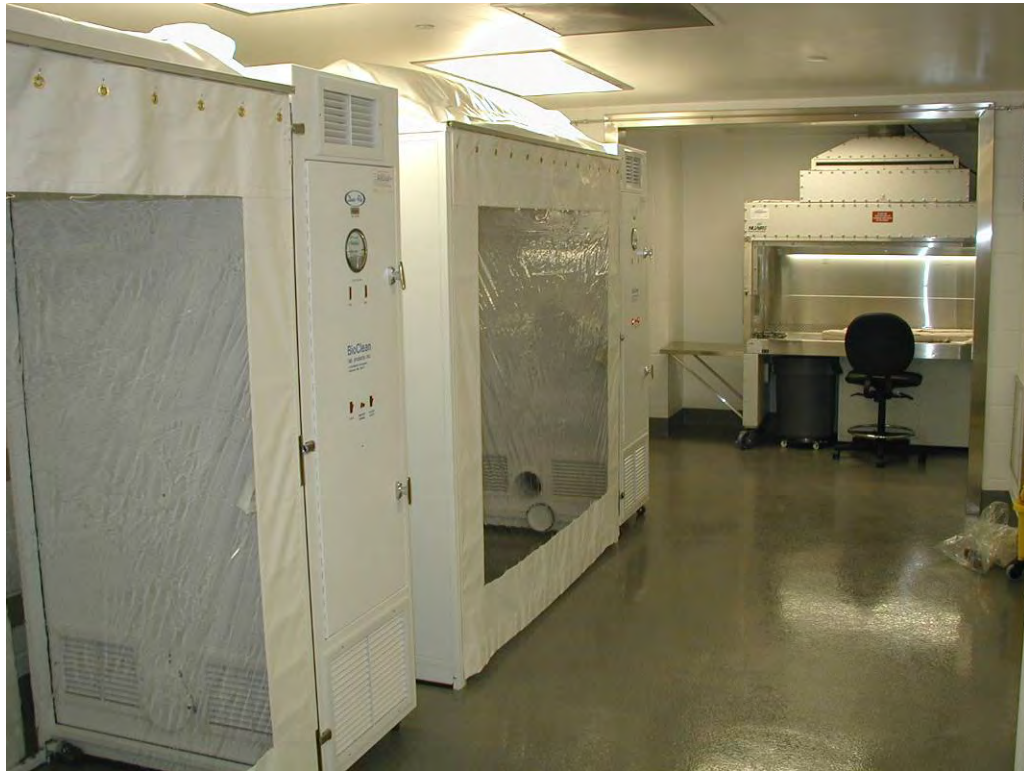
Portable isolators and change station
