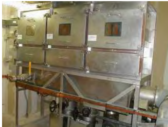
HEPA Exhaust with Decon Port
