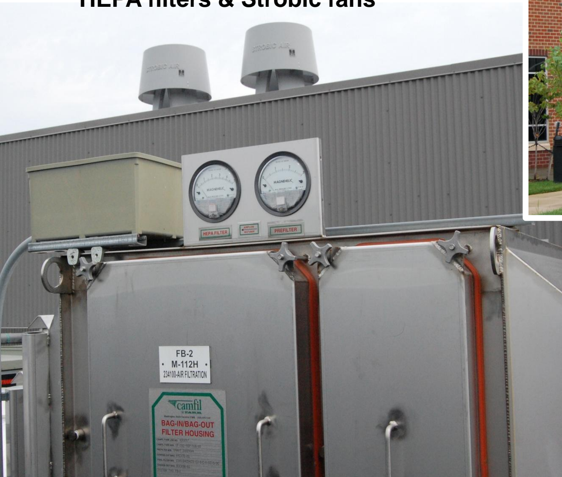
HEPA filters & Strobic fans
