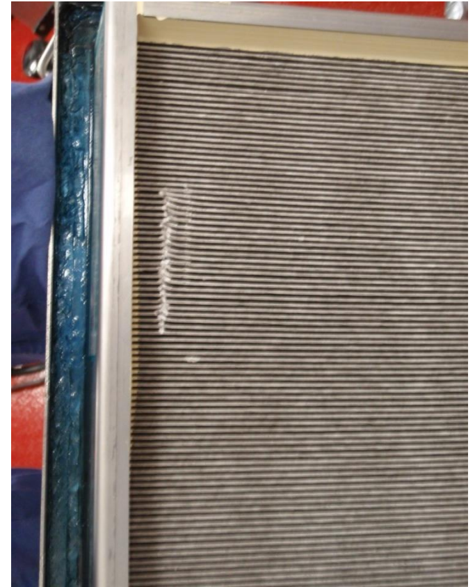
Damaged Supply Side Hepa Filter
