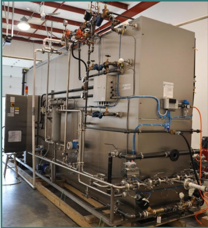
A large redundant 150 degree C system with regeneration
