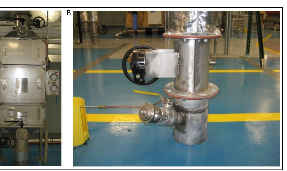
Figure 4. Decontamination ports on room exhaust HEPA filter housing (A) and room supply air (B).
