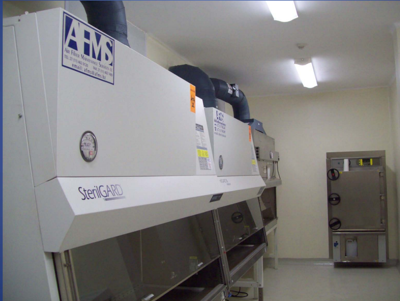
Certified BSCs and double-door autoclave
