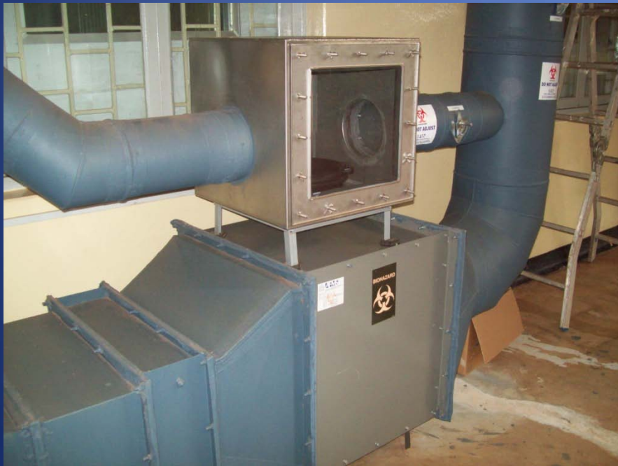
HEPA Exhaust System
