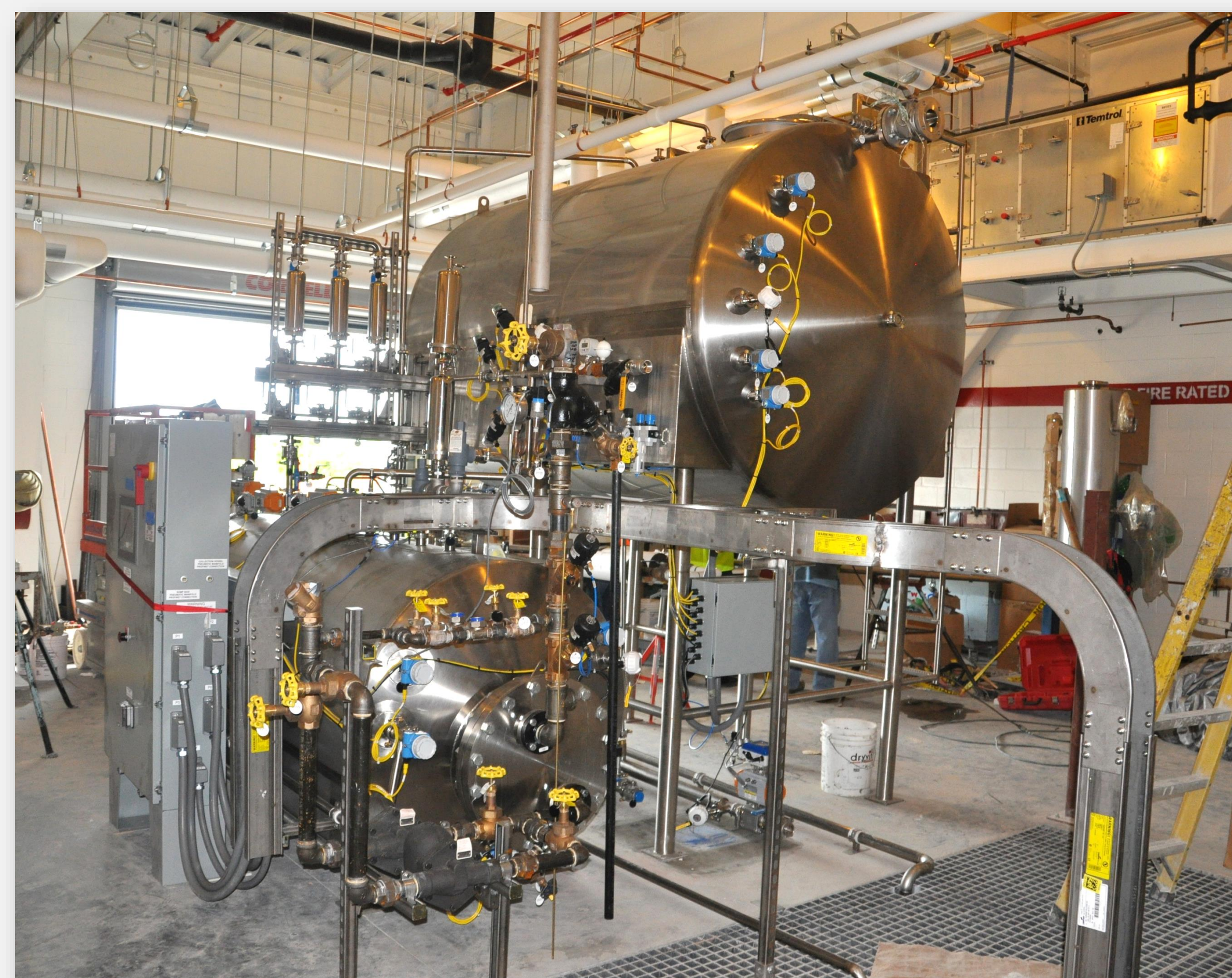
System above, 4 gpm continuous equivalent, capital cost $600,000, uses >20x more energy than the system at the right
