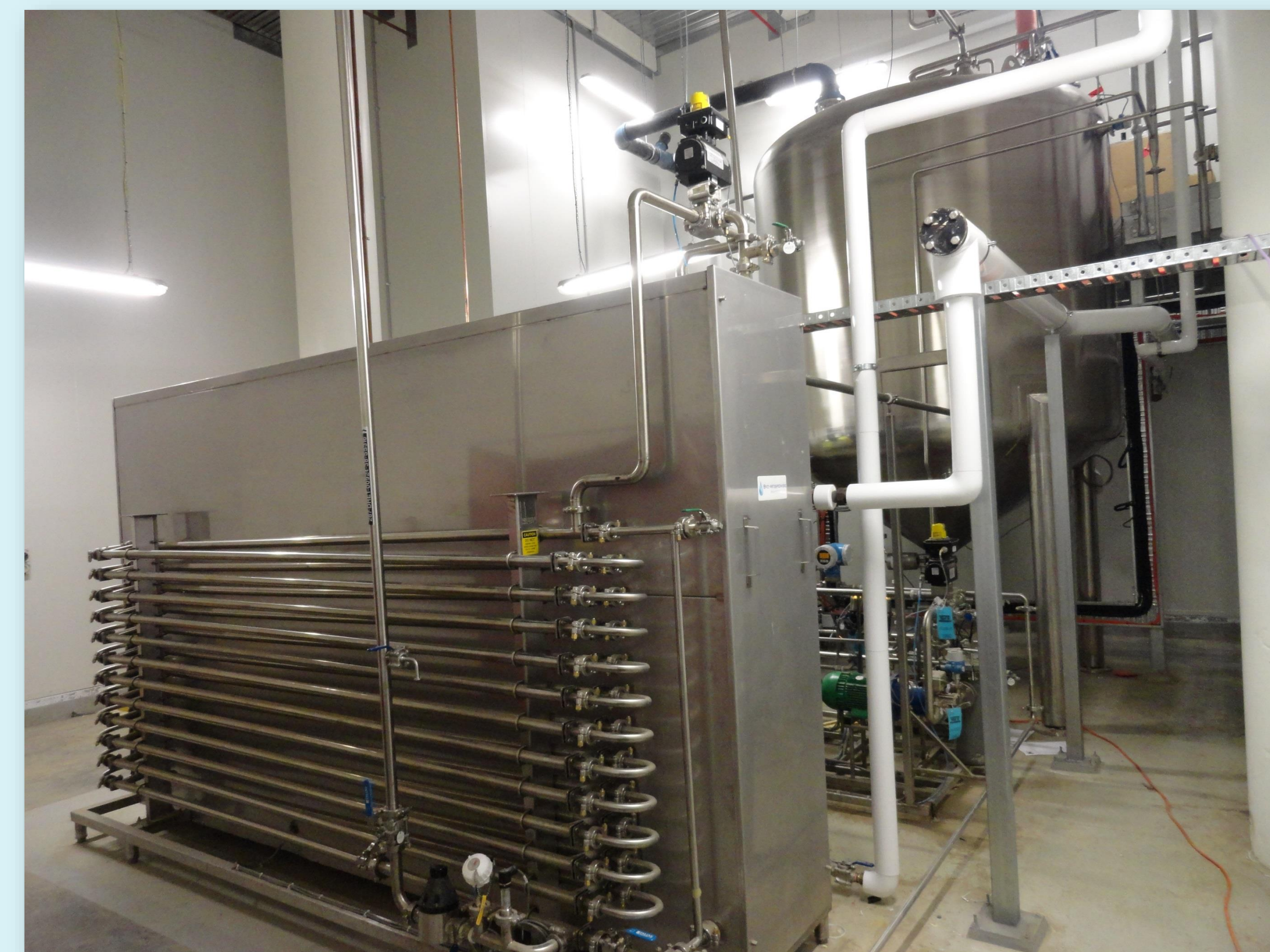
System above, 10 gpm continuous equivalent, capital cost $600,000, uses <5% of the energy of the system at the left
