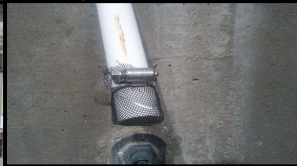
Insect netting on roof drain tubes
