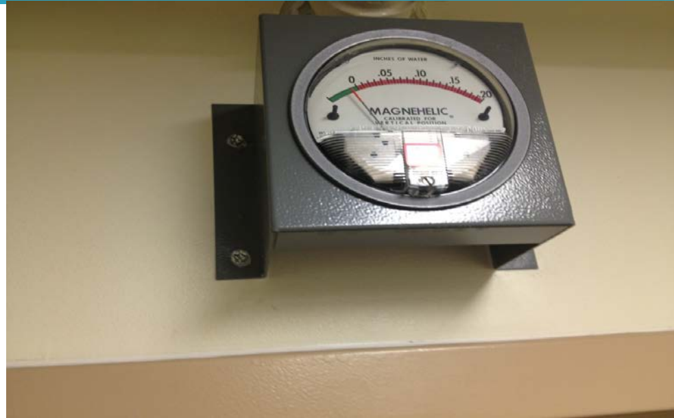
Magnehelic Gauges Read Neutral
