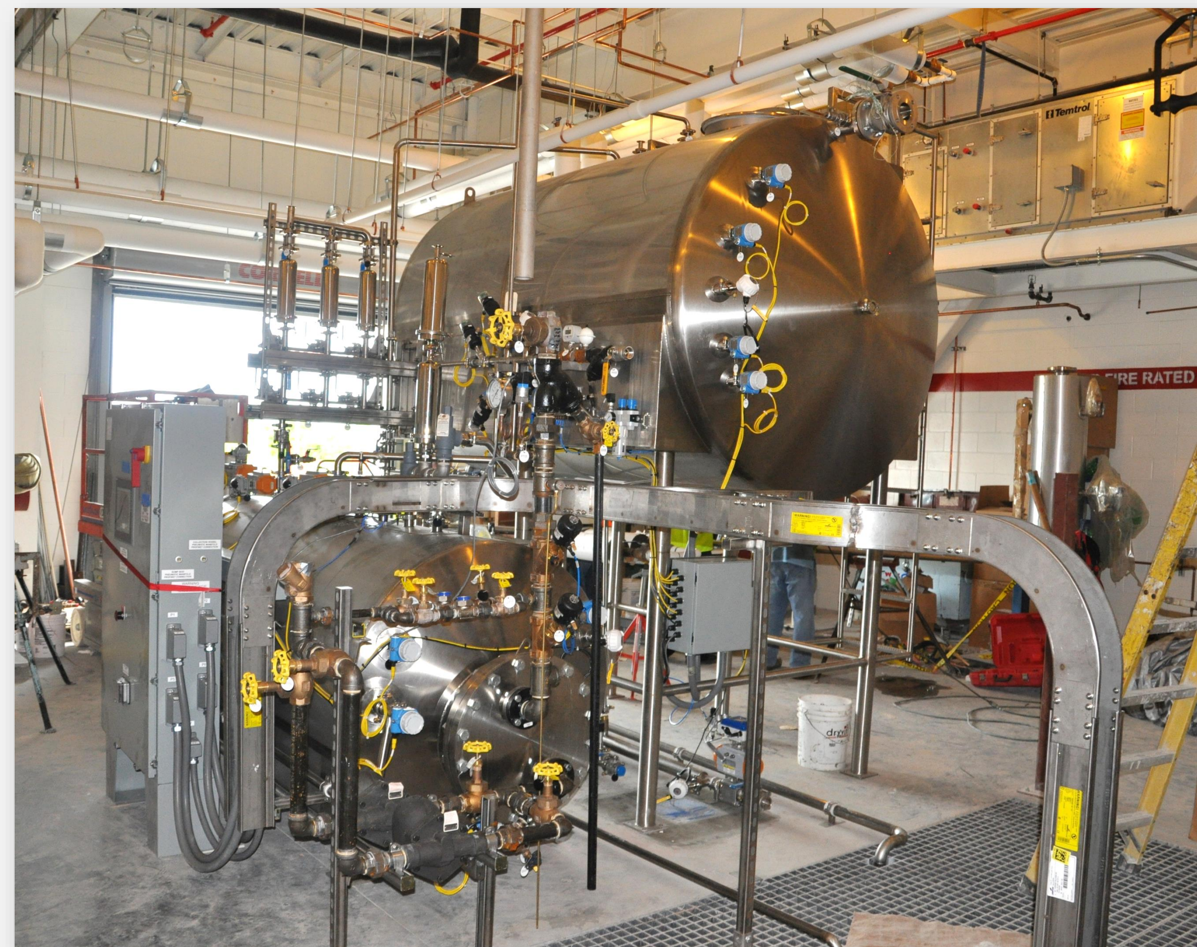
System above, 4 gpm continuous equivalent, uses >20x more energy than the system at the right; Higher Capital Cost!
