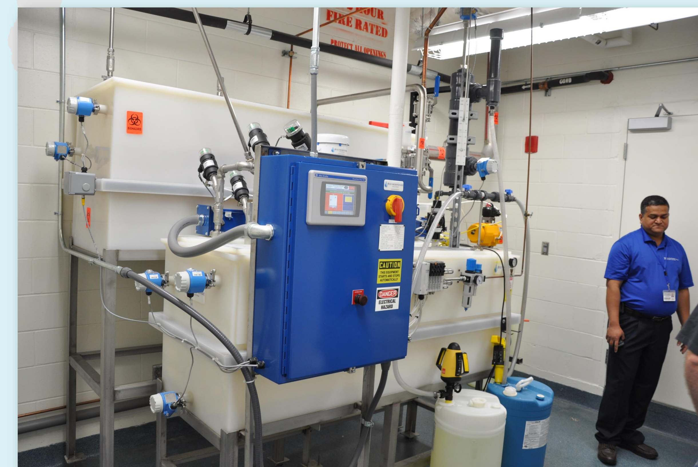
Batch Chemical EDS, 300 gallons per hour, $5 per hour ops cost, low capital cost
