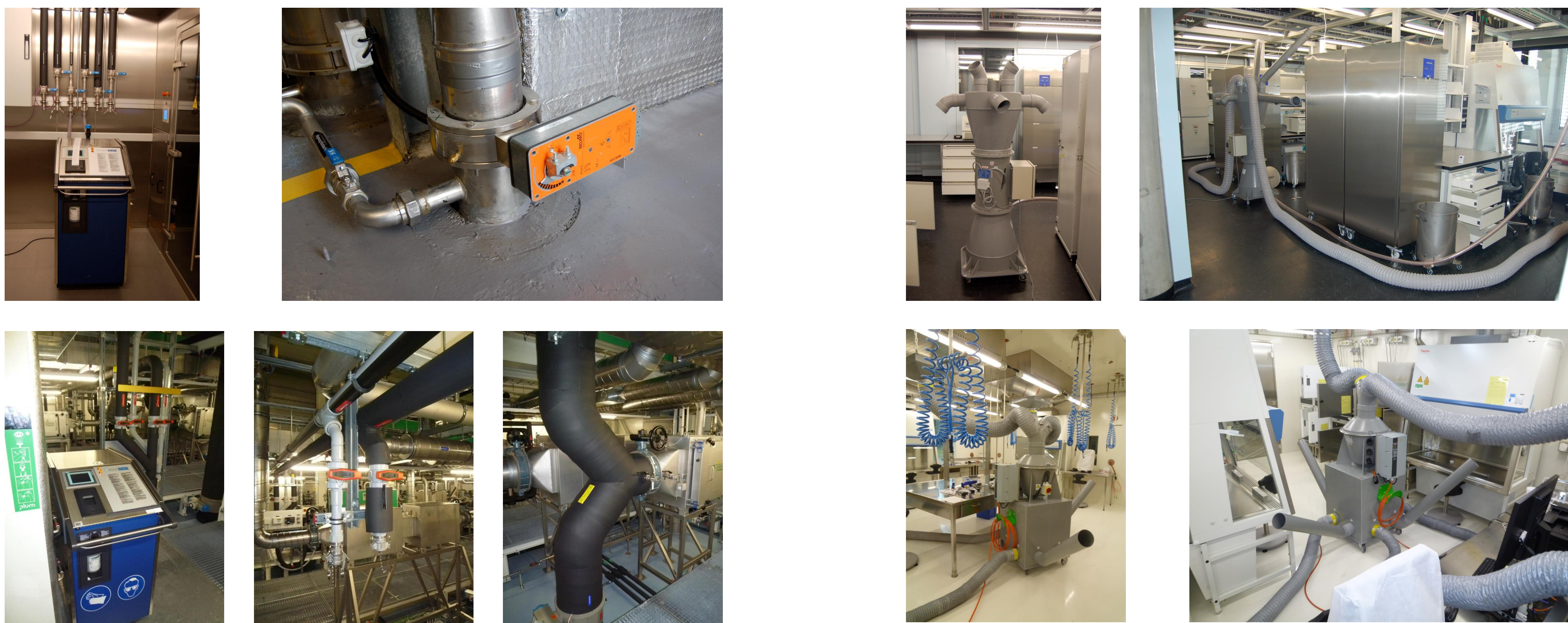
Figure 1: Bringing VHP into the fumigation zone is the first important step of any fumigation cycle. This can be done in different ways. The top pictures show a set up with dedicated fumigation lines leading directly into the room, while the bottom pictures show a distribution system leading into the supply air ducts. In both cases, insulation of supply lines is essential. However, smaller lines can be more easily pre-heated, thus reducing the risk of condensation. Supply air ducts may be more difficult to pre-heat and often require additional heating on besides insulation. In this case supply air ducts were additionally fitted with heating coils to achieve higher surface temperatures in the ducts in order to control condensation.
